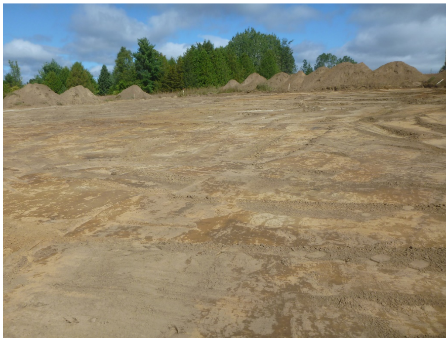
Image 5: The Duncan Site (BfGd-9) following mechanical topsoil removal, view west.
