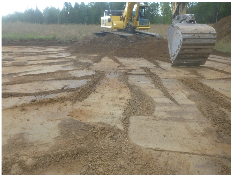
Image 3: Excavator conducting mechanical topsoil removal, view west.
