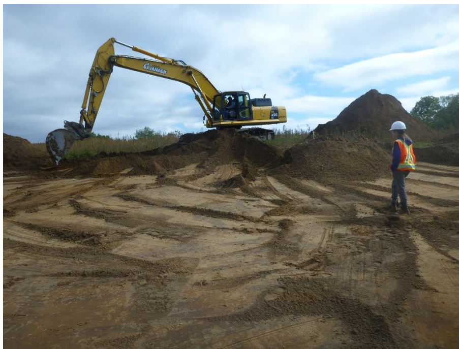
Image 4: Excavator conducting mechanical topsoil removal, view northeast.
